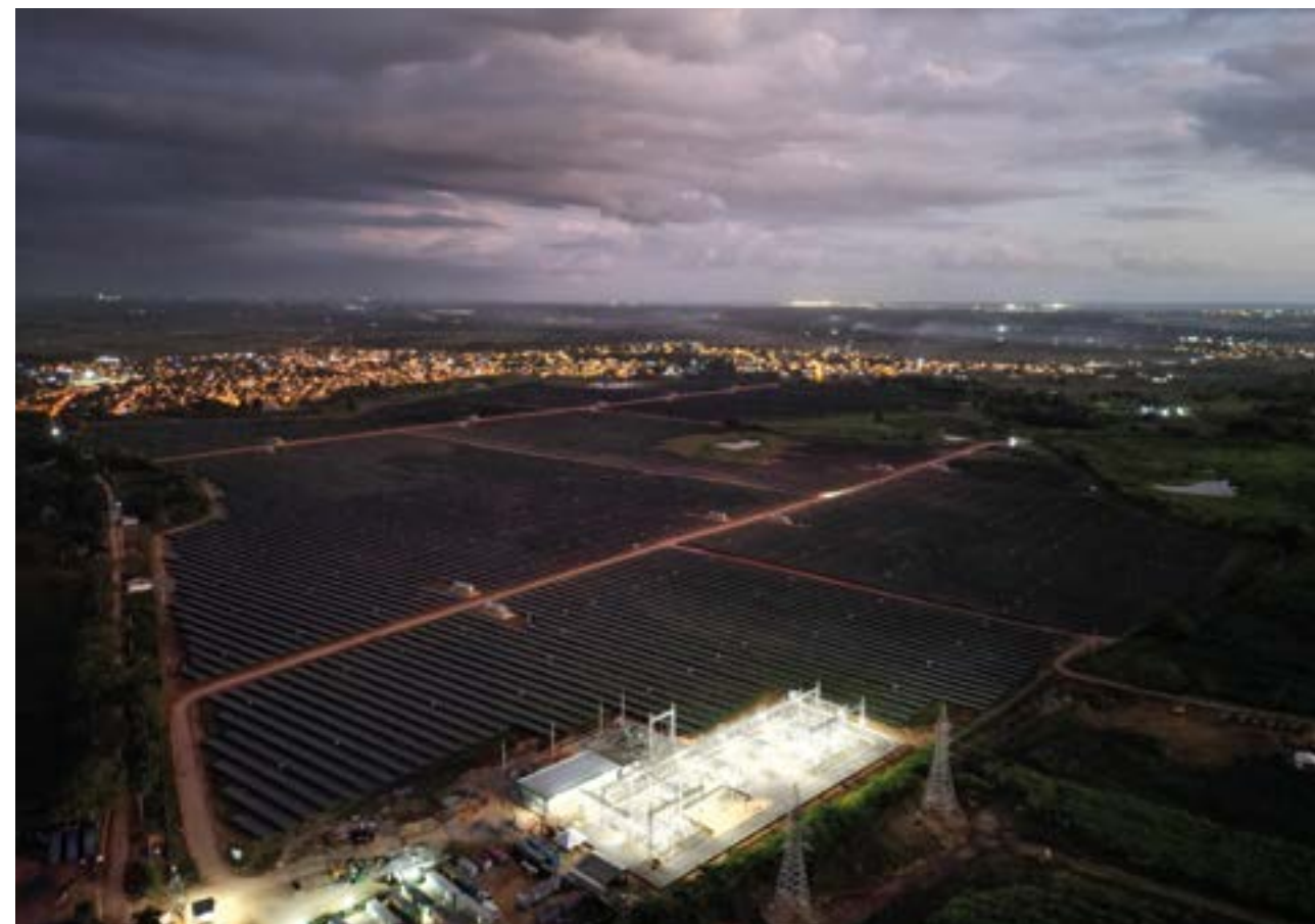
MIRASOL 127 MW PHOTOVOLTAIC PLANT + SE + LT (DOMINICAN REPUBLIC)
