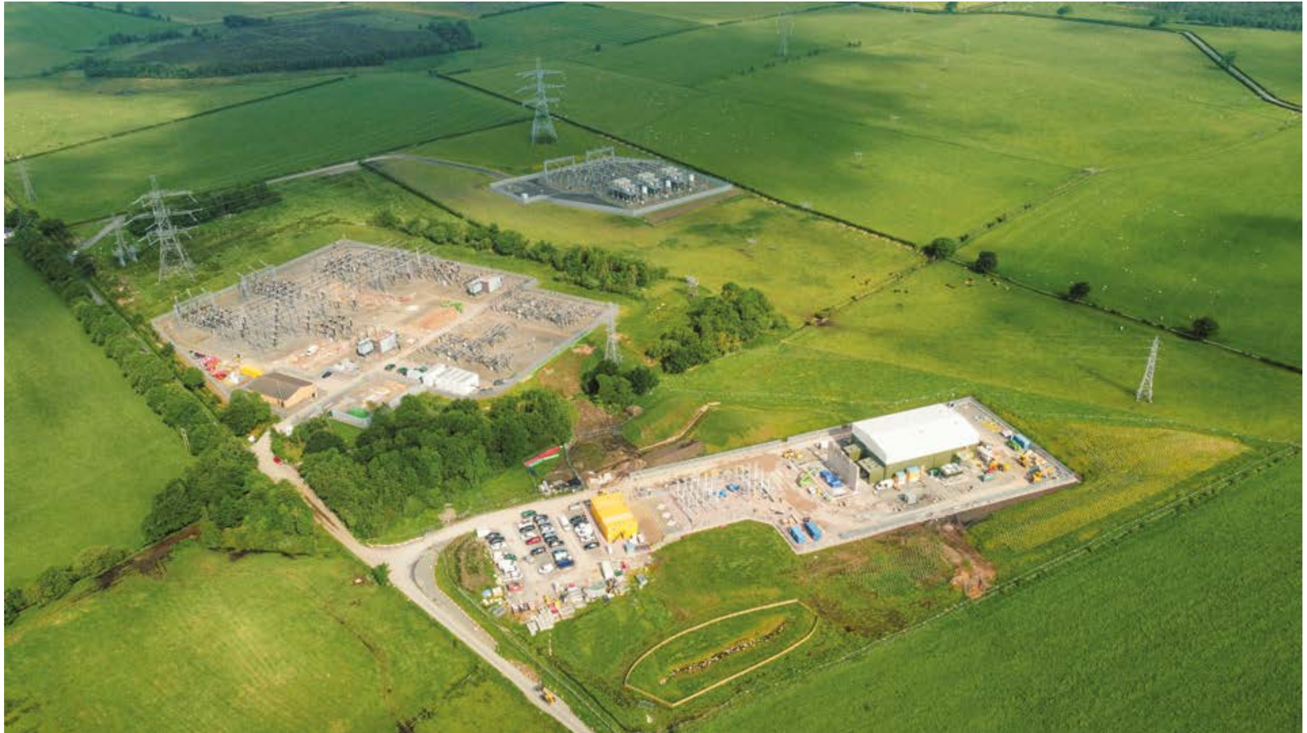
GRID STABILITY PLANT GREтна (UNITED KINGDOM)
