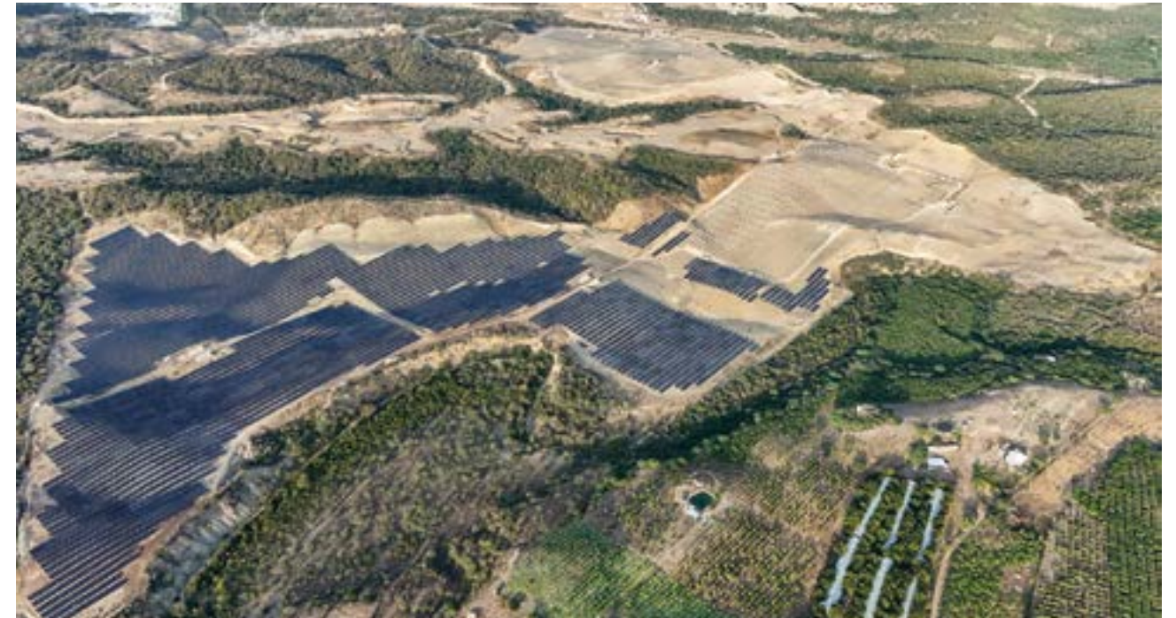
PERAVIA I AND II PHOTOVOLTAIC PLANTS 180 MW (DOMINICAN REPUBLIC)
